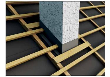
For maximum waterproofing we recommend using an appropriate roofing sealant where the sides of the chimney flashing meet the tiles and also where the chimney flashing connects to the chimney wall.
