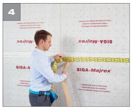
Seal overlap with Sicrall avoiding tension and wrinkles
