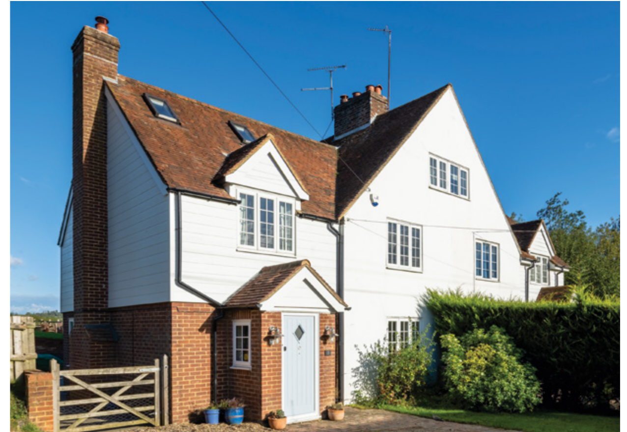
Hardie® VL Plank cladding installed horizontally – Colour: Arctic White
